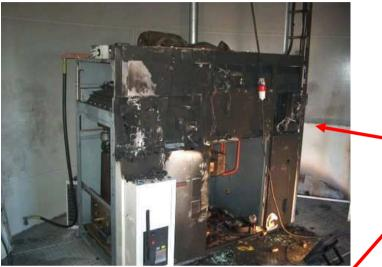
OVERVOLTAGE: short circuit in one electrical panel. Source: bad connection on one power cable lightning Estimated claim: 45.000 EUR + BI
