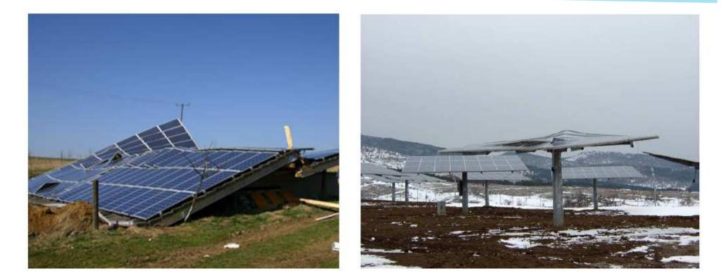
Storm damaged modules - demonstrate that many plants were not capable of withstanding the occurring exposure.
